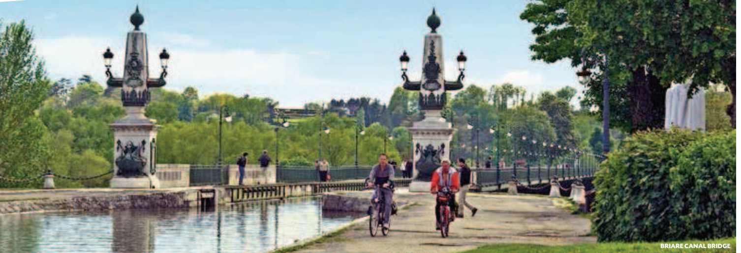
BRIARE CANAL BRIDGE
